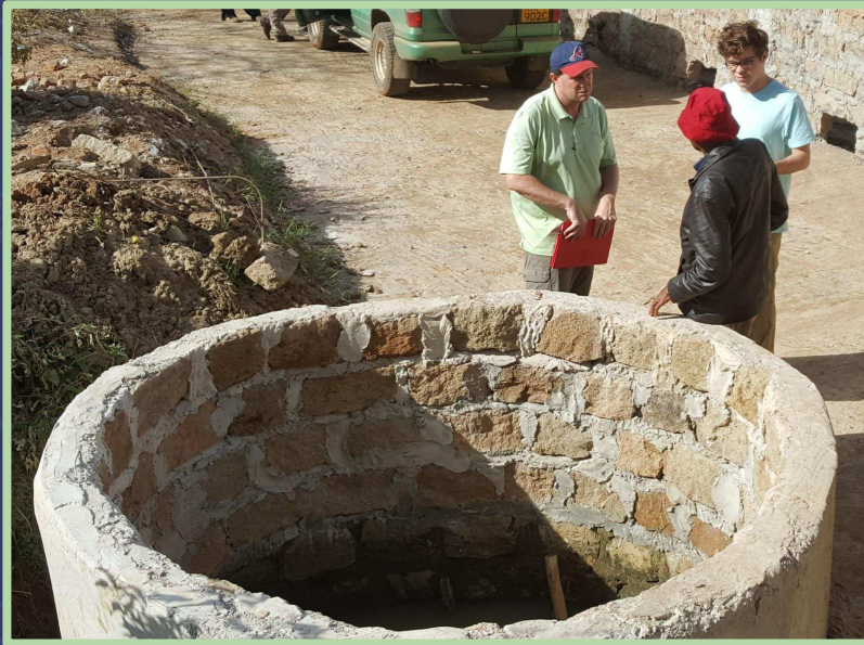
(Left) Aerial view of Mountain View property at MITS with completed wall around compound. (Middle) Completed well which will use solar powered pump.
