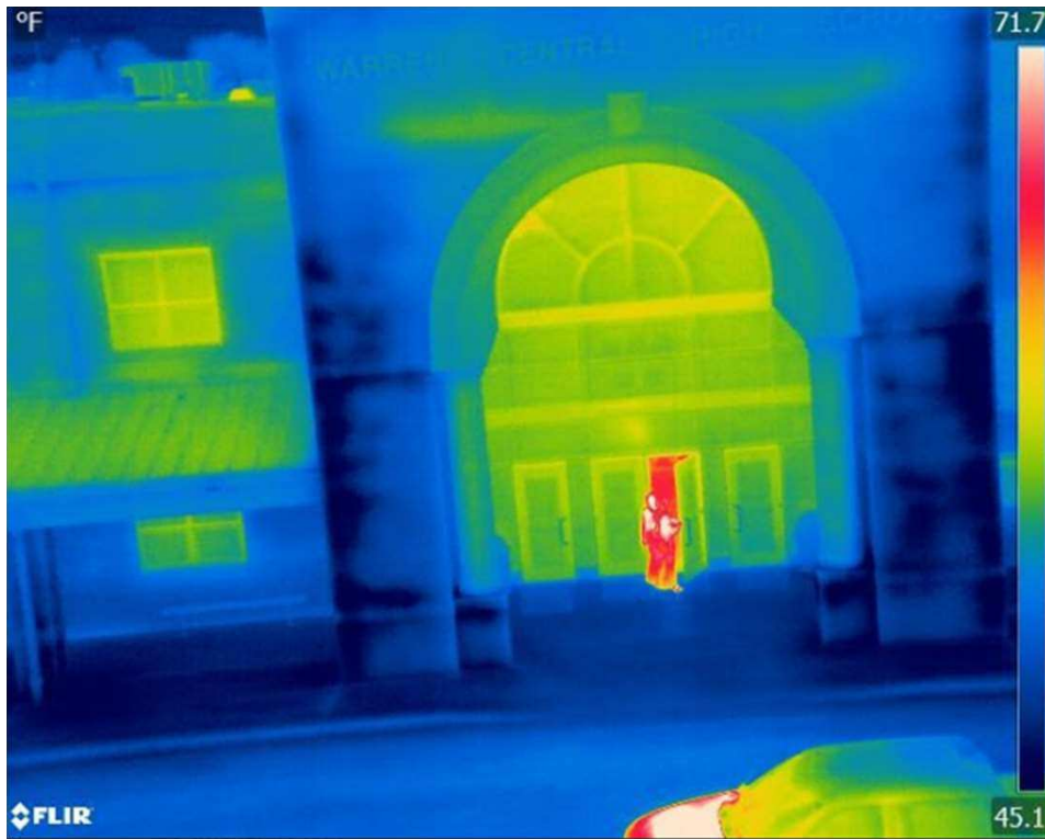
Thermal image of front entrance of school
